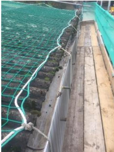
Figure 1. An example of a suitable perimeter scaffold to which the nets are tied
